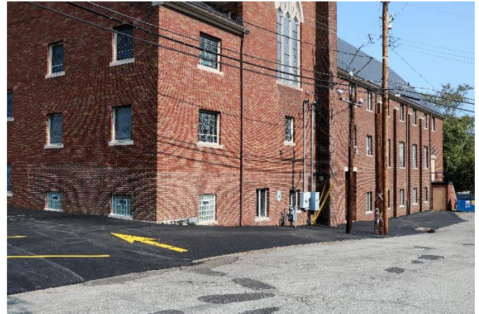
Our newly paved James Street Entrance
