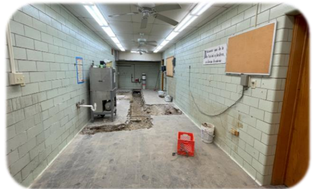
Kitchen floor, counters, & appliances removed & trench dug to replace plumbing
